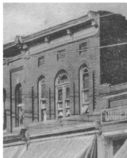
Historic cornices of 5 N. Water
