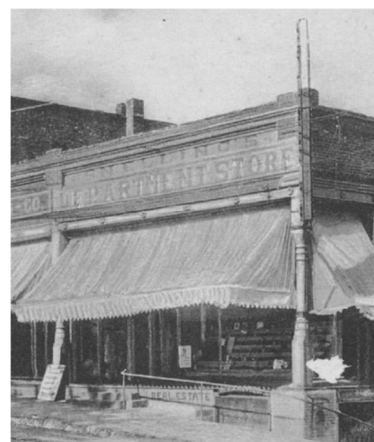
Original brick relief and pilasters
