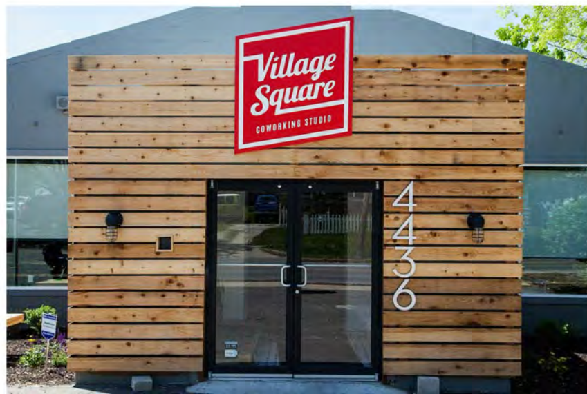
Example of reclaimed wood veneer
